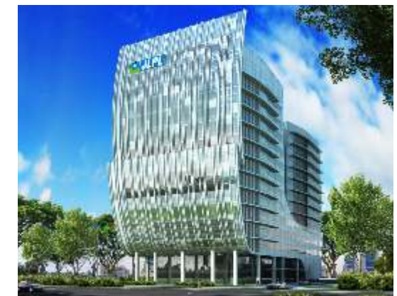
IT Twin Towers Sector 66-A
